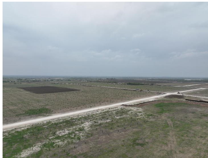
SOLAR FARM Midlothian, Texas
