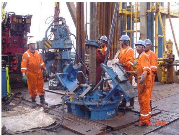
Tubing Hanger Mode Instalation
